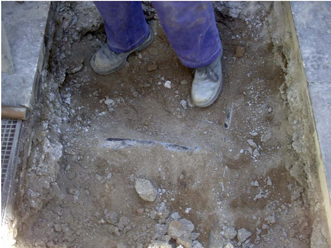
Foto 6: Rasa 2, carrer Veguer.
